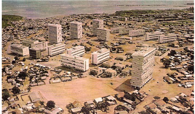
Figures 1 and 2 - Neighborhood Unit number 1: project model and construction
