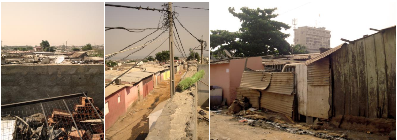
Figures 15, 16 and 17 – Materials and construction quality of self-construction houses. Various aspects.
