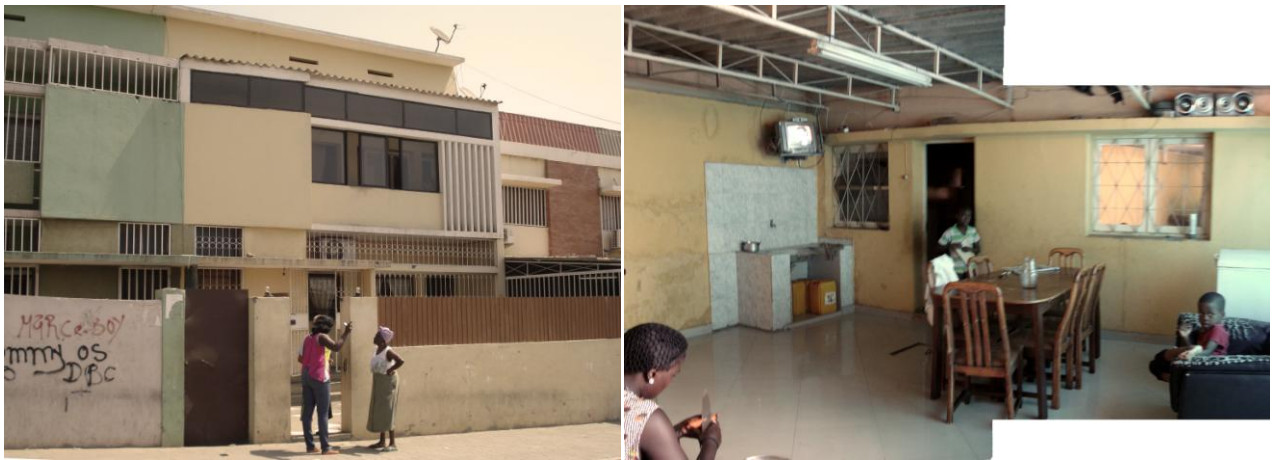
Figures 7 and 8 – Visited townhouse, main façade and new kitchen.
